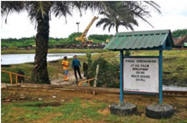
Water discharge point for Effluent Waste Water Treatment
