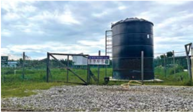
Water Treatment Plant (Poh Zhen Plantation)
