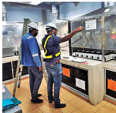
On-site LEV inspection
