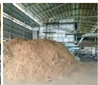
Mill boiler with Press Fiber as bio-fuel.
