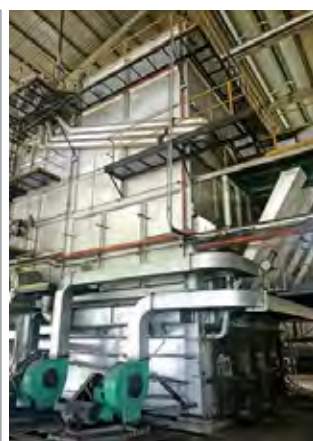
Mill boiler with Press Fiber as bio-fuel.
