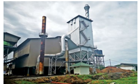
ESP system (Wealth Houses CPO Mill)
