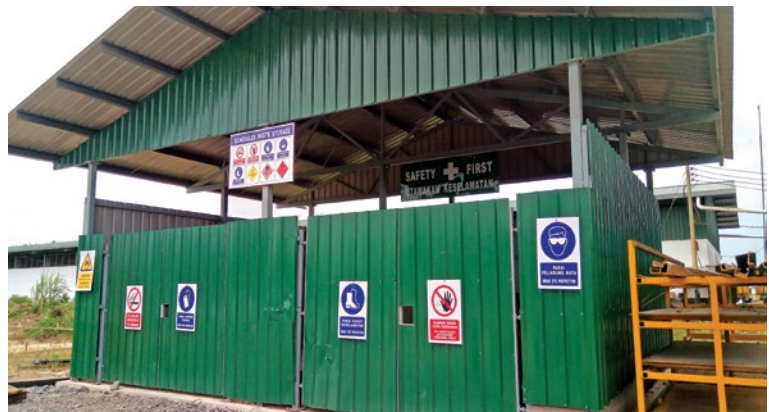
Scheduled Waste Store
