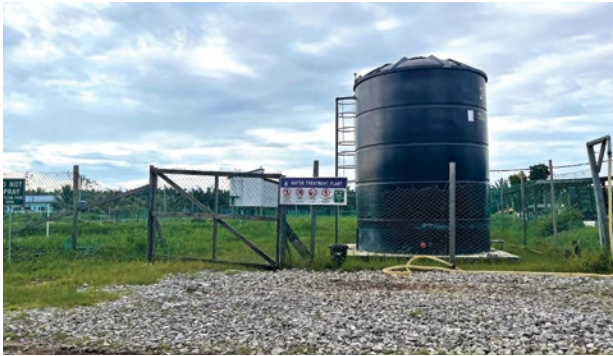
Water Treatment Plant (Poh Zhen Plantation)
